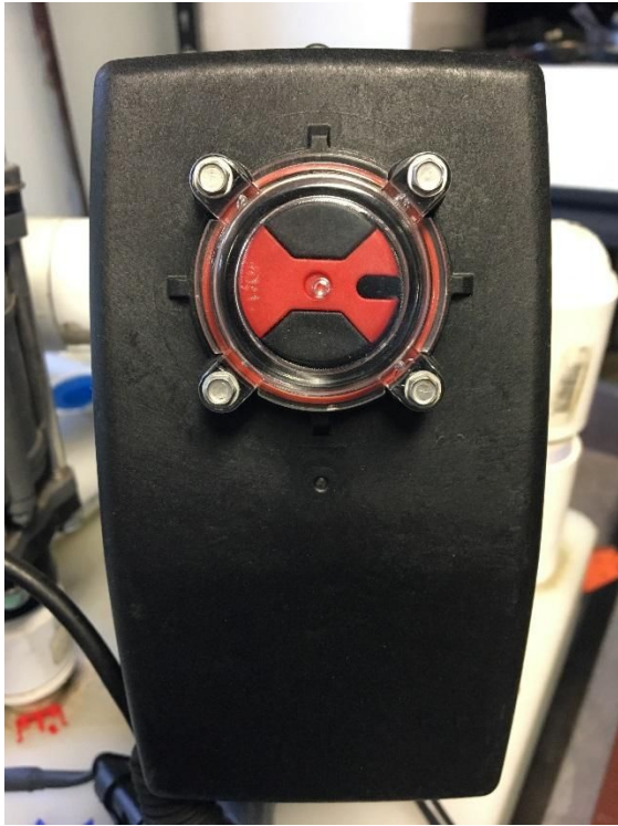
Figure 4: Control Valve - NOTE: Red indicator shows valve position, photos show valve in Closed Position ↓ (i.e ➡ = Open Position in the above photos and ↓ = Closed Position)
